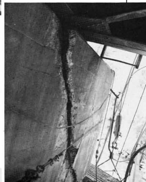
Problem on D&RGW bridge in Colorado: severe split in its second pier.
