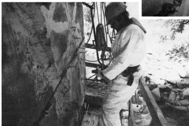
Osmose technician injecting epoxy formulations to 'weld' crack shut.
