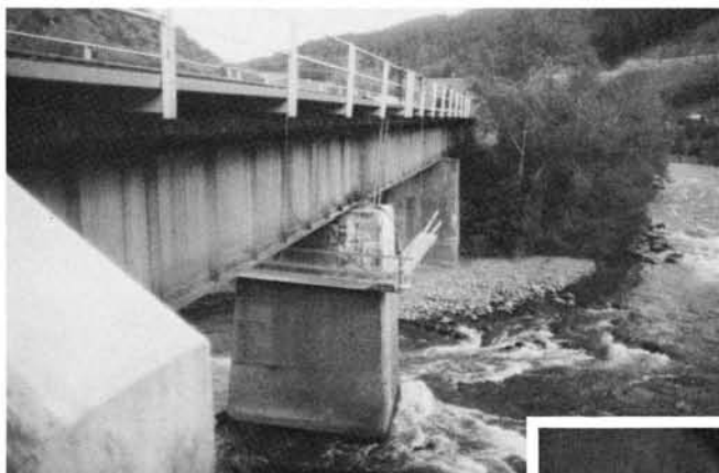
Problem on D&RGW bridge in Colorado: severe split in its second pier.
